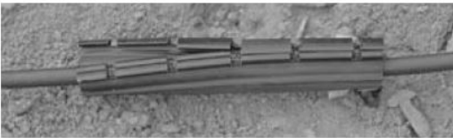
2. Wrap sleeve around connector and shut snap locks over entire length of sleeve.
